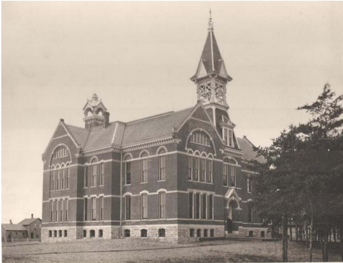
MARINETTE—HIGH SCHOOL BUILDING.
